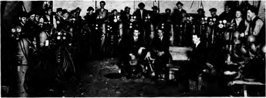
Group of Brown Brothers' welding operators, showing the extent to which this young business has grown.
